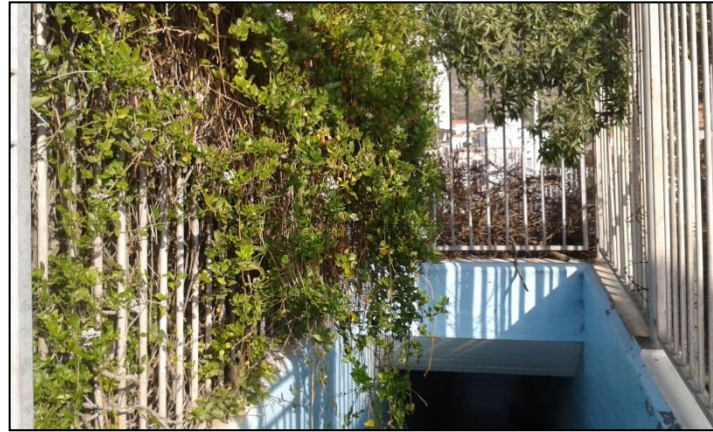
Figure 5: Overhanging branches that will be trimmed near the church road subway.
