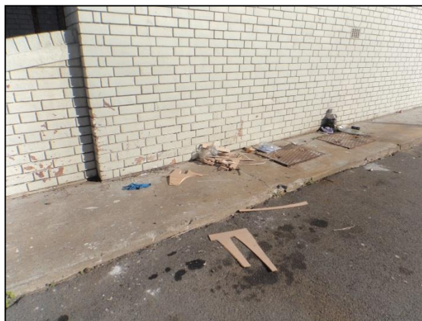
Figure 2: An area used by street people unfortunately results in a build-up of litter.
