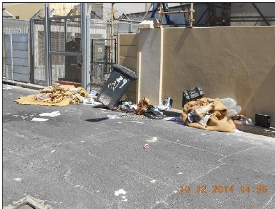
Figure 8: Waste collection site after the municipality emptied the refuse bins. Many items were not taken.
