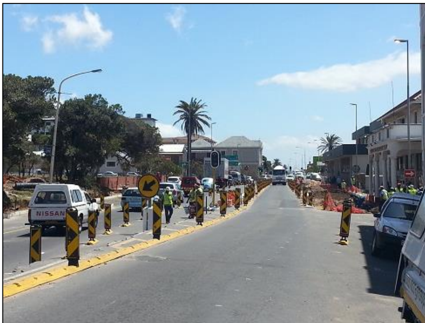
Figure 5: Road maintenance on Main Road.
