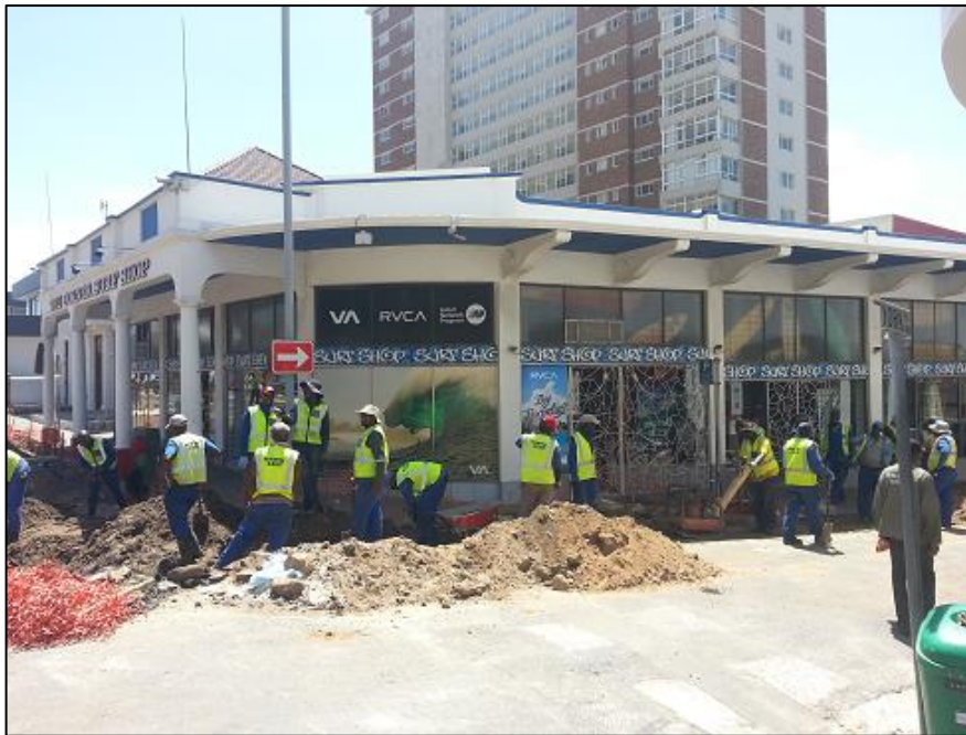
Figure 6: Road maintenance on York Road
