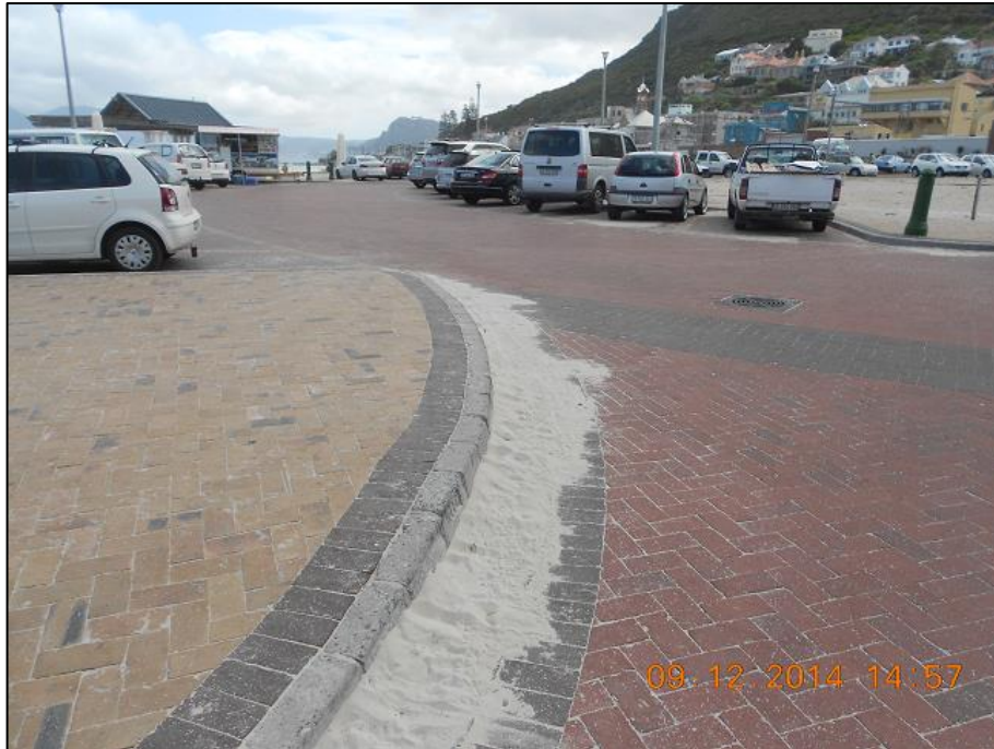
Figure 3: Sand build-up at Surfers Corner.
