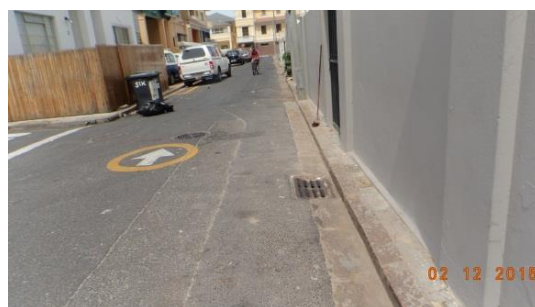
Figure 3.b. Church street after.
