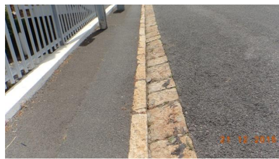
Figure 7.b. Gutter cleared of weeds.
