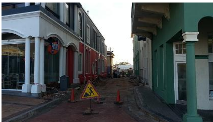
Figure 2: Roadworks in Sidmouth Road.
