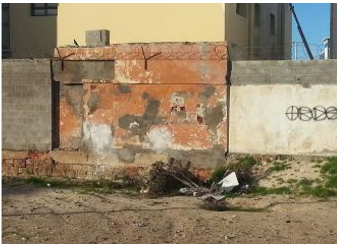
Figure 16: More waste dumped on the corner of Church and Alexander Road.
