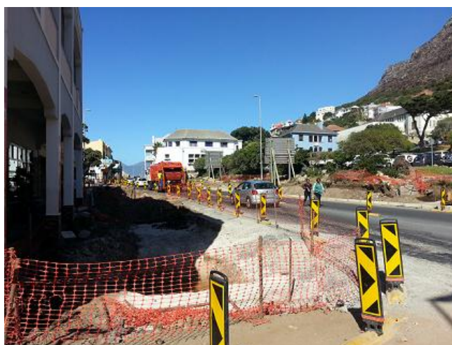
Figure 5: Roadworks in Main Road.
