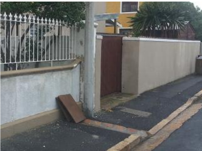
Figure 14: Boards dumped in Holland Road.
