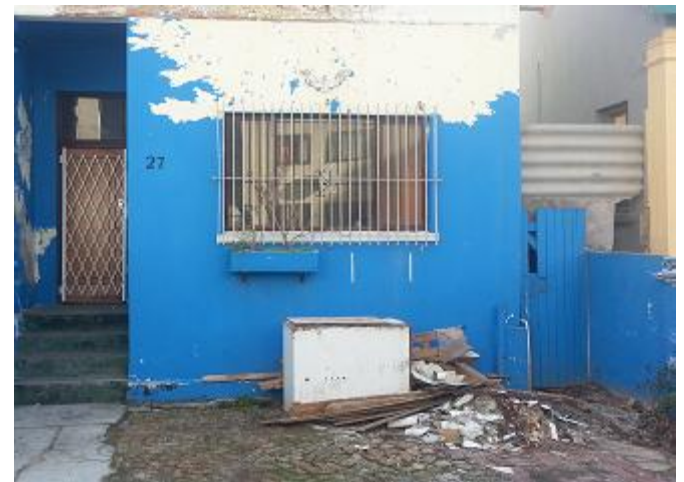
Figure 15: Builders rubble dumped in Church Road.
