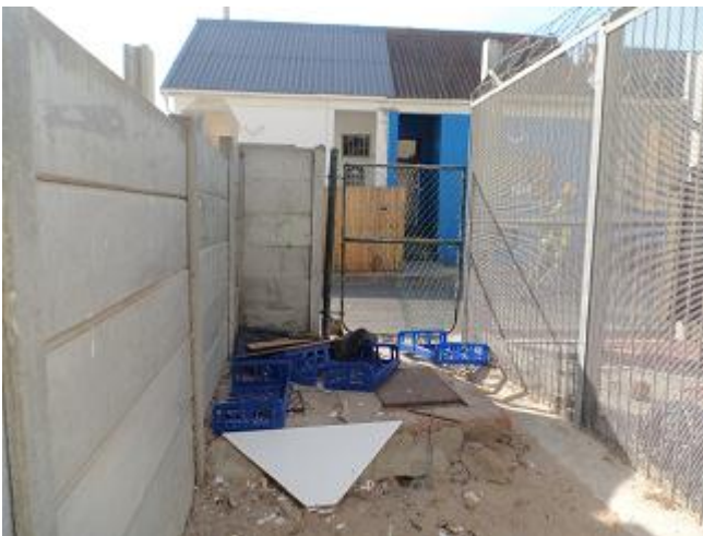
Figure 14: Dumping in the vacant area next to the transformer in Church Street.
