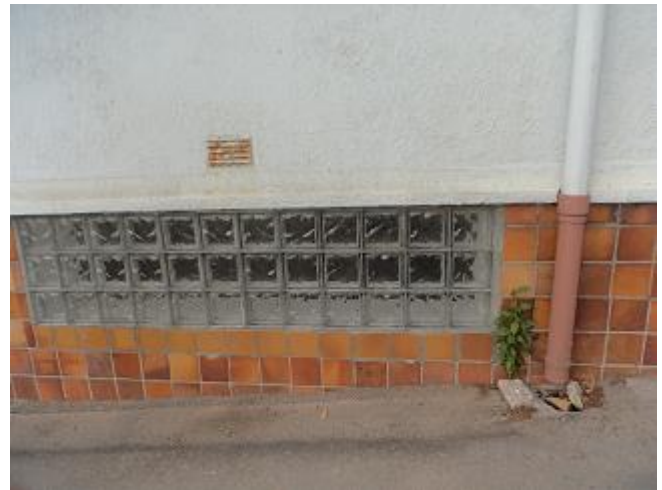
Figure 10: The area in figure 9 after being cleaned.
