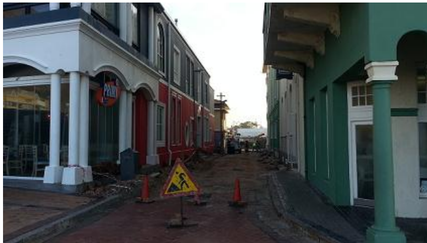
Figure 8: Roadworks in Sidmouth Road.
