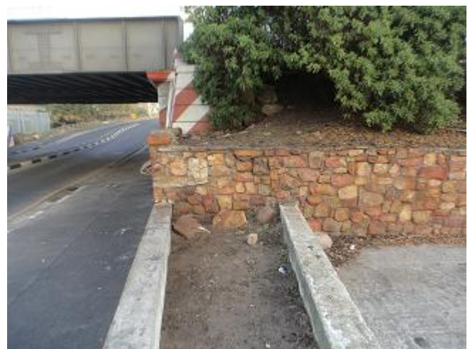
Figure 5: The area in figure 4 after being cleaned.
