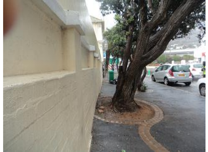
Figure 7: The area in figure 6 after being cleaned.
