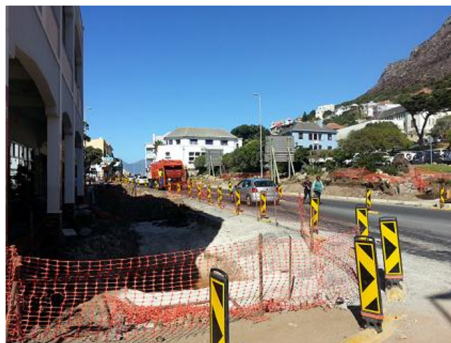
Figure 11: Roadworks in Main Road.
