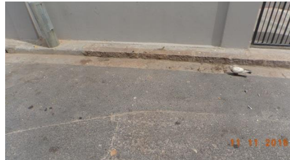
Figure 2.b. Church road After
