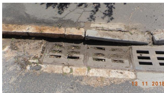
Figure 5.b. Gutter cleared of weeds.
