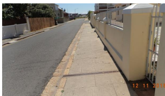
Figure 4.b. Pavement walls cleared of weeds.
