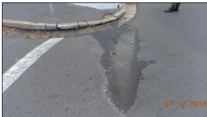
Figure 9: One of the leaking valves on the corner of Palmer and Holland road.
