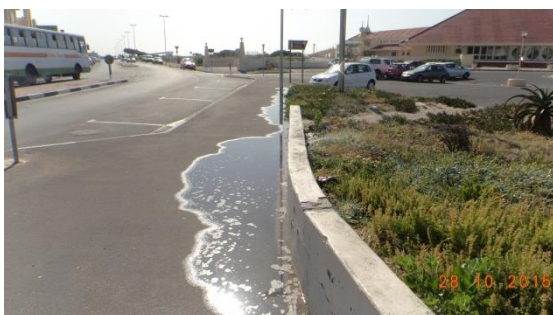
Figure 14.a. Irrigation leakage.
