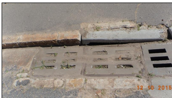
Figure 10: One of the blocked drains in Albertyn road.
