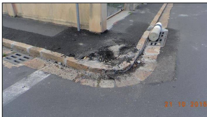
Figure 8: The broken bollard.
