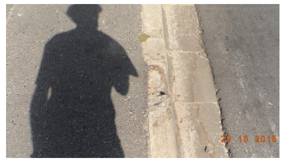
Figure 16.b. Fractured kerb stones .
