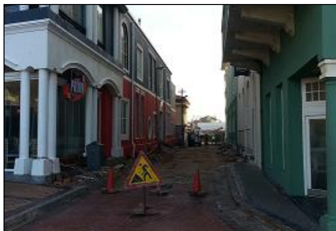
Figure 3: Construction underway in Sidmouth Road.
