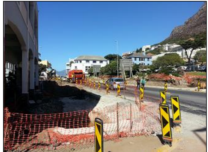
Figure 5: Road Maintenance activities on Main Road.
