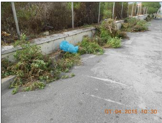
Figure 11: The fence after all the overgrown vegetation had been trimmed
