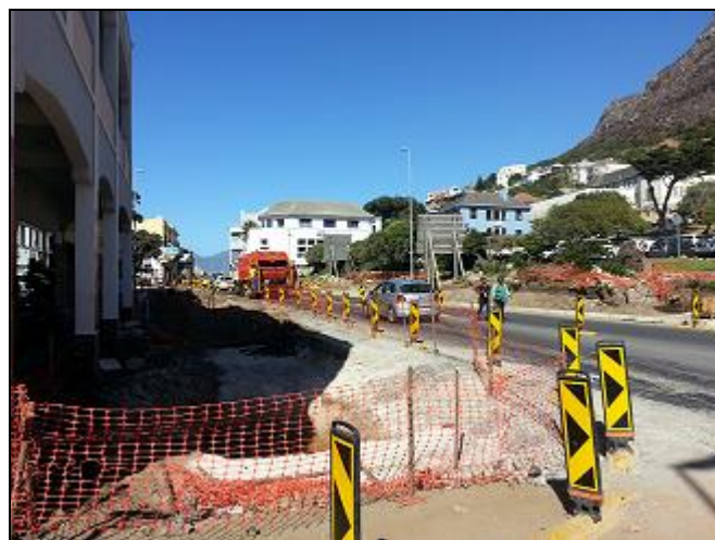
Figure 5: Road Maintenance activities on Main Road.
