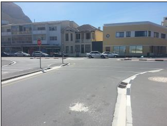
Figure 2: Sand build-up in the road gutters on the corner of Beach and Atlantic road.
