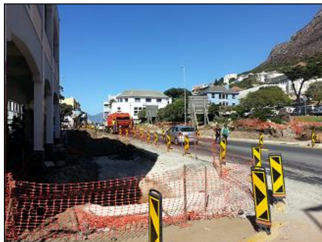
Figure 4: Road Maintenance activities on Main Road.
