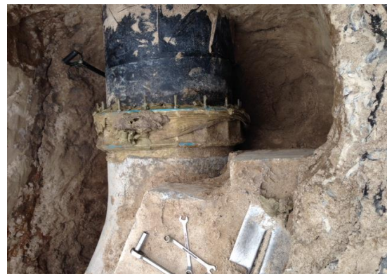
Example of typical mechanical coupling
