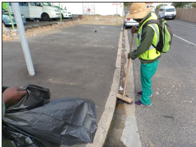
Figure 6: Servicing of guttering system on Main Road and Belvedere Road.
