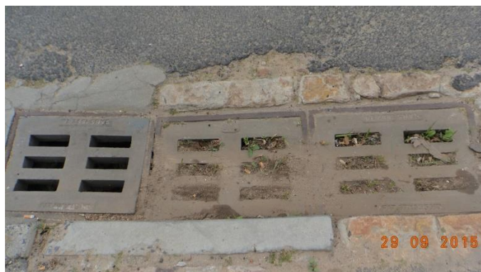
Figure 3 and 4: Due to the flooding that occurred in August 2015, most drains in Rhodesia road is blocked and filled with sand and to be addressed.
