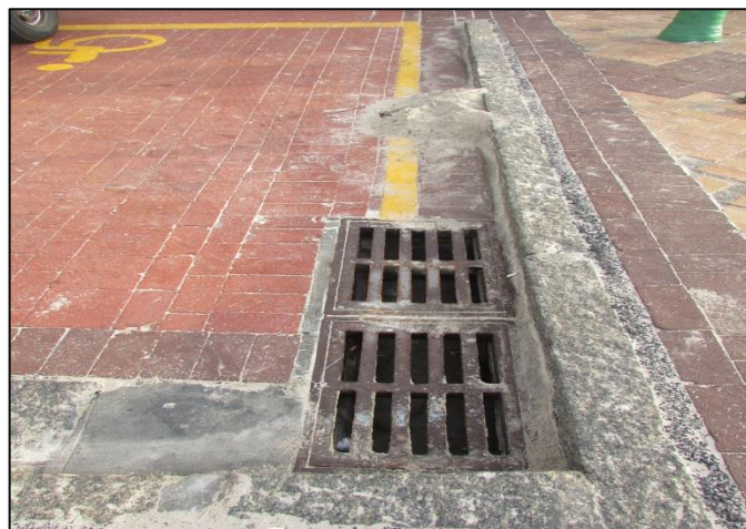
Figure 2: Maintenance of guttering system at Surfers Corner Parking Area.
